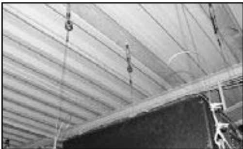
Figure 15: Eyebolts in place of threaded rod
